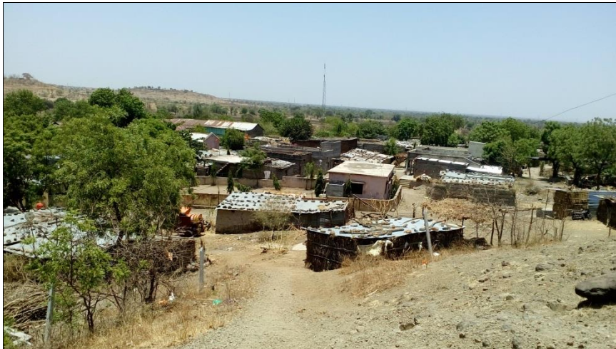
Photo2: Tin roof households in the villages
