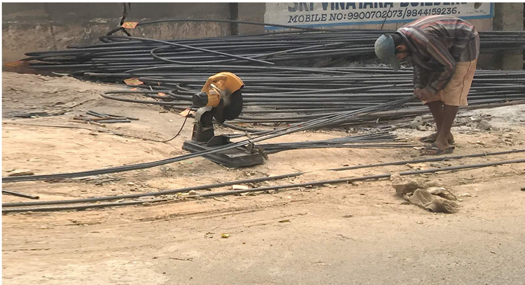
Construction workers cutting steel rebar for the building foundation, all under the watchful eye of the foreman.
